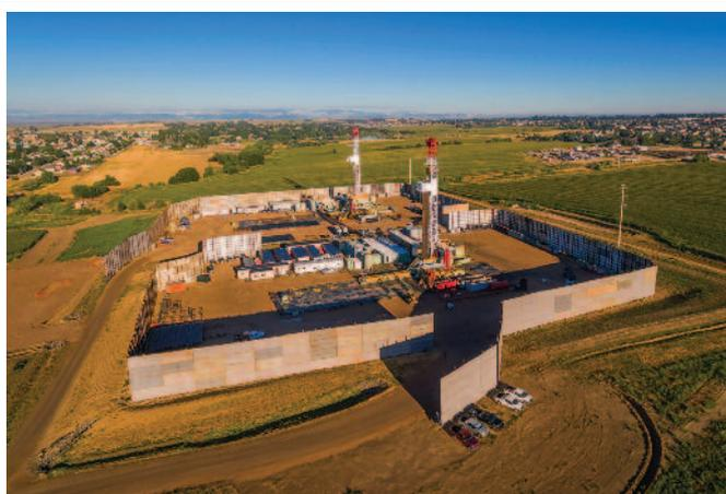
Temporary 32-foot sound walls enclose SRC Energy Inc.’s Evans pad in the D-J Basin, dramatically reducing noise and light output from wellsite operations. The two rigs finished drilling 22 horizontal wells on the pad last year, including 13 ‘long-length’ laterals averaging 10,000 feet and nine ‘extended-length’ laterals averaging 12,000 feet. Ahead of the horizontal drilling program, SRC plugged 27 legacy vertical wells on the Evans spacing unit and reclaimed
